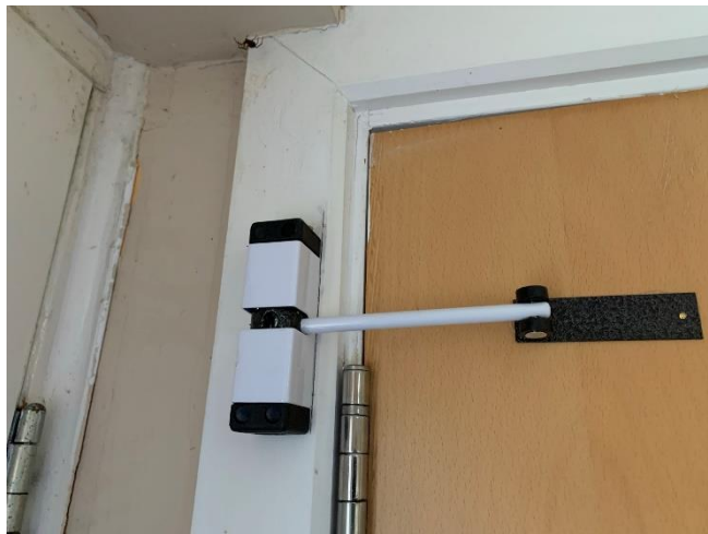
Potentially unsuitable closer device
