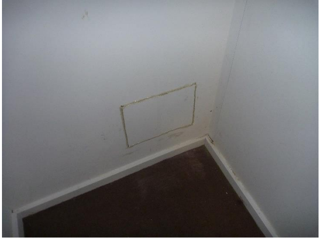
Damaged wall with foam used as repair
