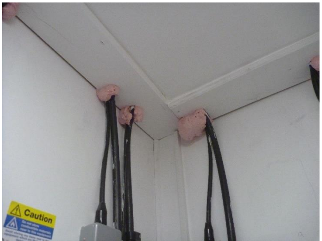
Damaged wall with foam used as repair
