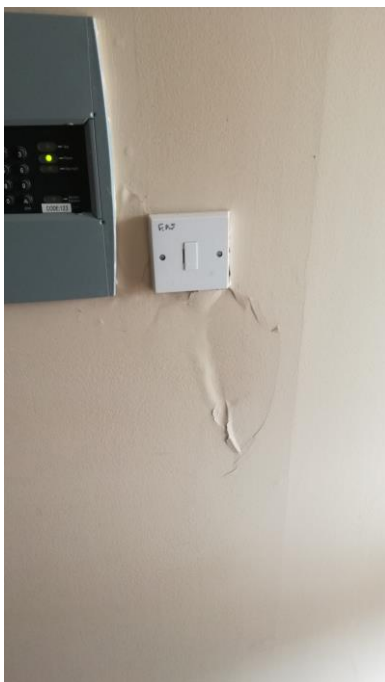
Damaged plasterboard
